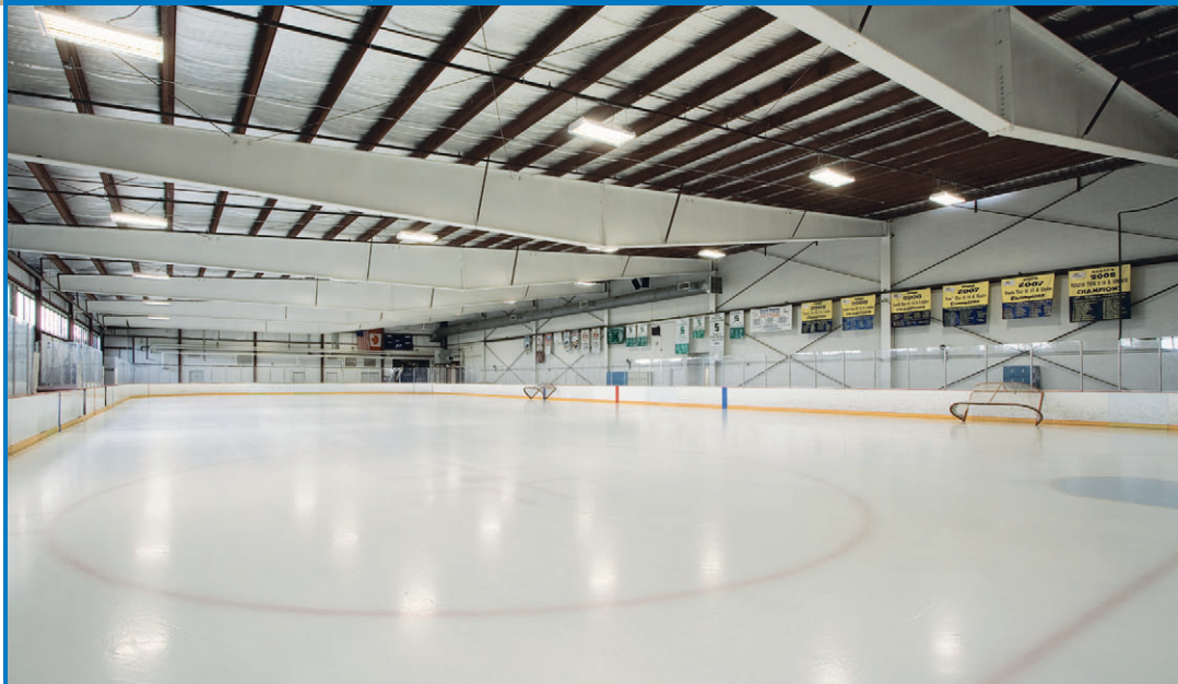
Dwyer Arena, Auxiliary Ice Arena—After
